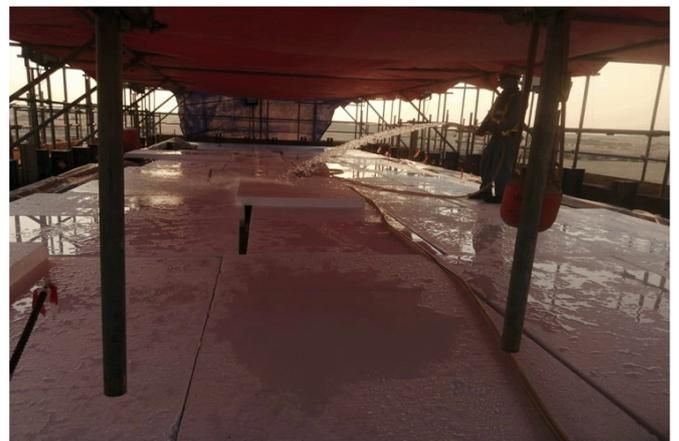
**Figure 1:** Insulation, Water Curing and Shading as Mitigation Measure for Compressor Mass Foundation No. 1
